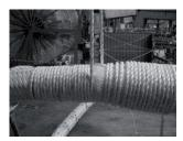
Pull the seizing with a lifting device. If there's no lifting device present, pull the seizing after each winding tied by hand.
