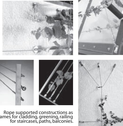
Rope supported constructions as frames for cladding, greening, railing for staircases, paths, balconies.
